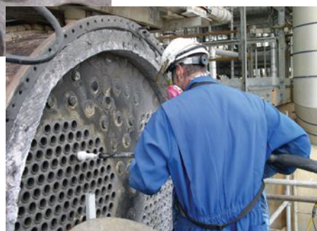
NitroLance™ cleaning Frontier's waste heat boiler.
