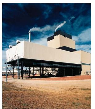
Fig 4. Air Cooled Condenser in Black Hills Plant
